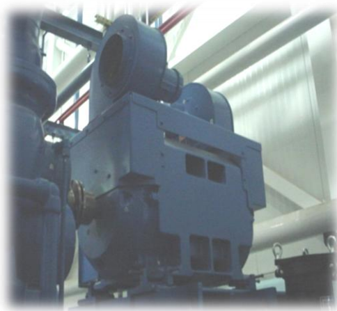
500 HP inverter rated motor (North Ice Cream Plant)
